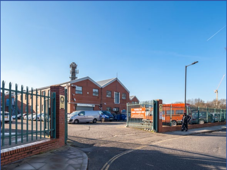
Burgess Business Park entrance
